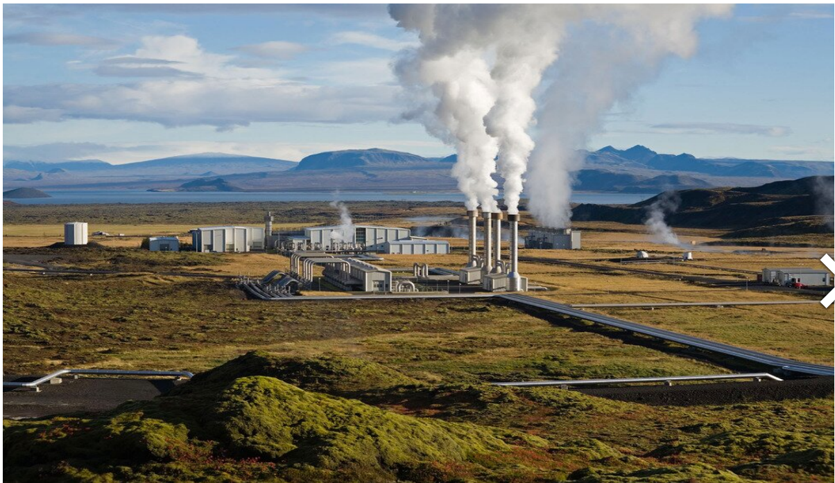
Geothermal power plant
